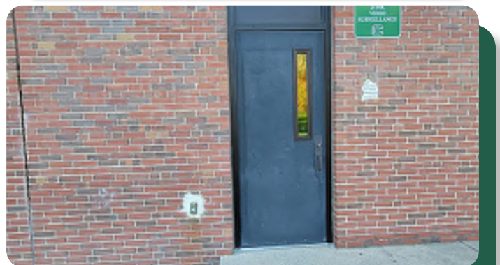
Typical exterior service door showing some fading
