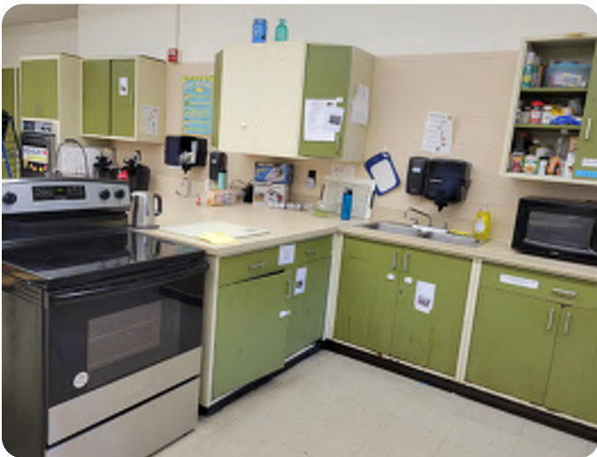
Life Skills classroom has original casework
