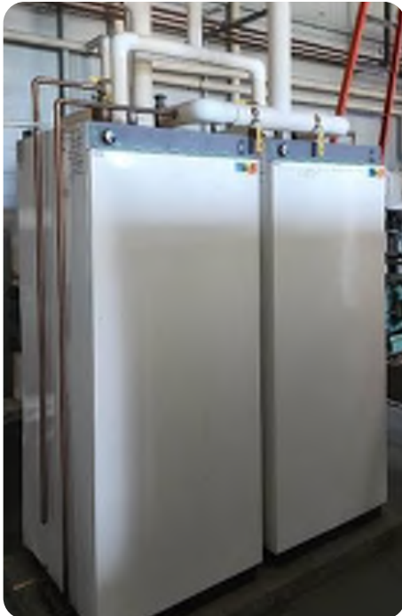
Indirect Water Heaters
