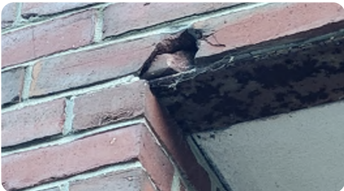
Damaged brick
