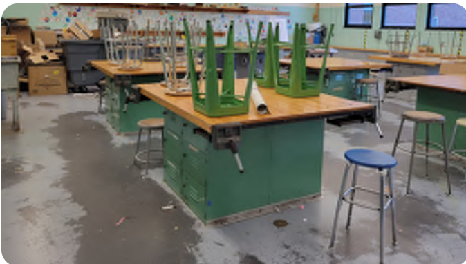
Painted concrete floor in Tech Ed. classroom
