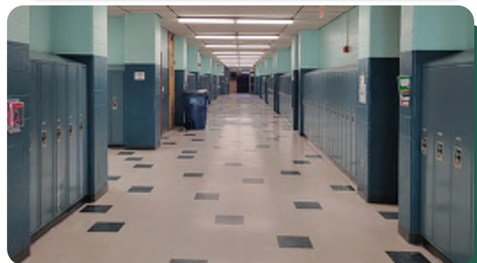
Typical academic corridor with CMU walls & lockers
