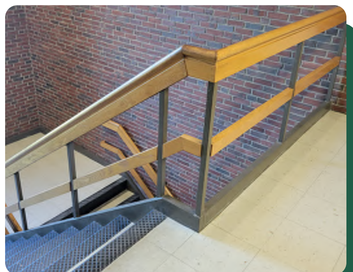
A 4" sphere can be passed through the stair rails
