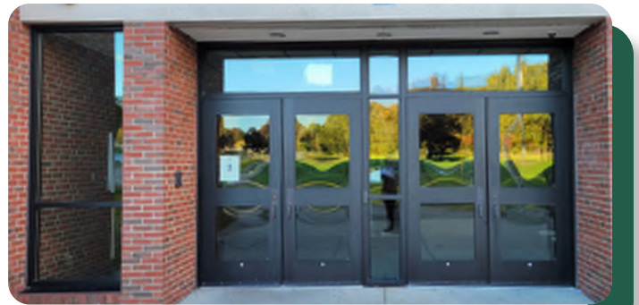
Replacement window and doors at main entrance
