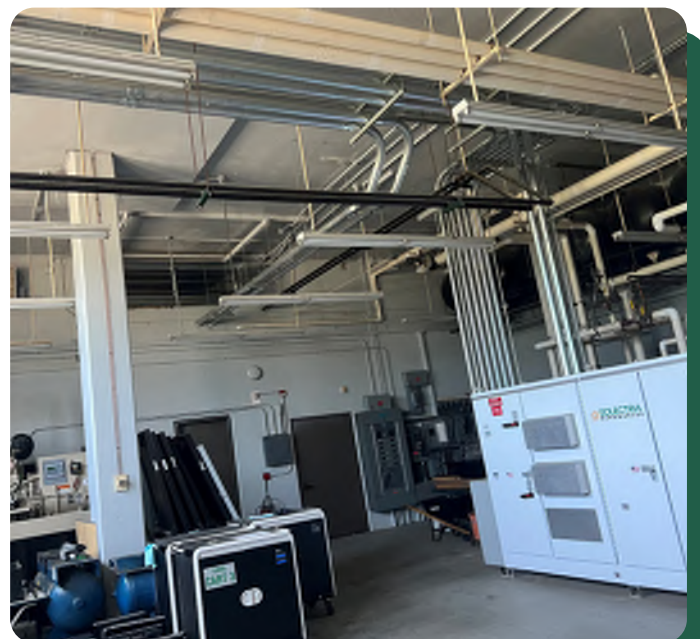
Typical floor slab viewed from Mechanical room
