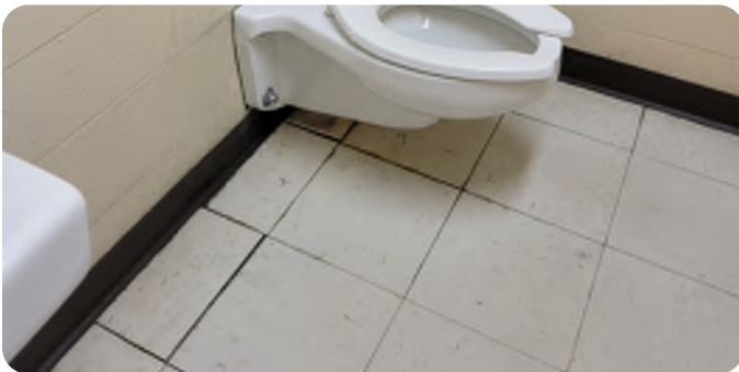
Lifting VAT in toilet room
