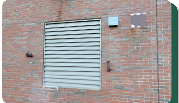
Mechanical louver in good condition
