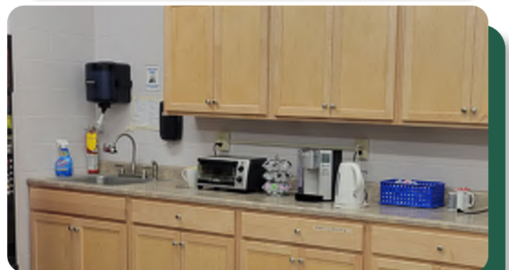
Office sink that does not meet accessibility req's
