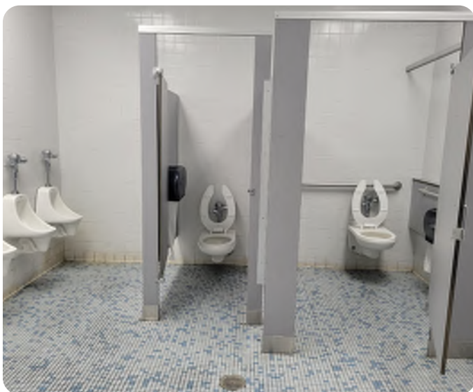
Typical toilet room interior
