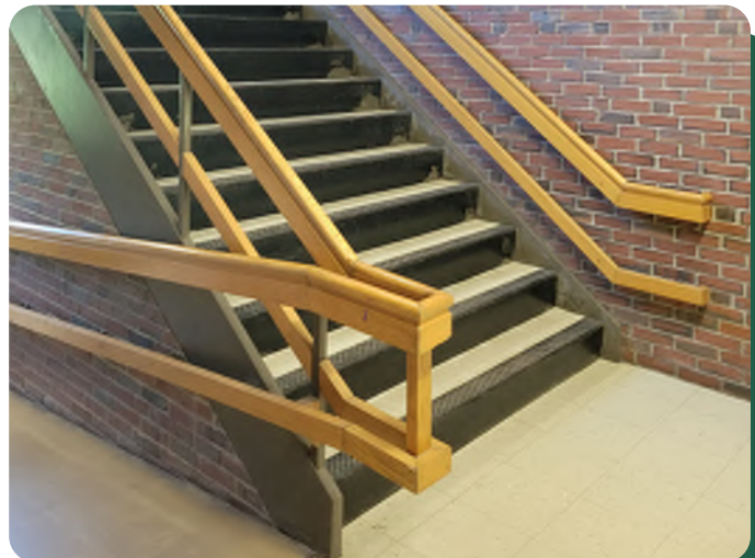
Existing stair railings
