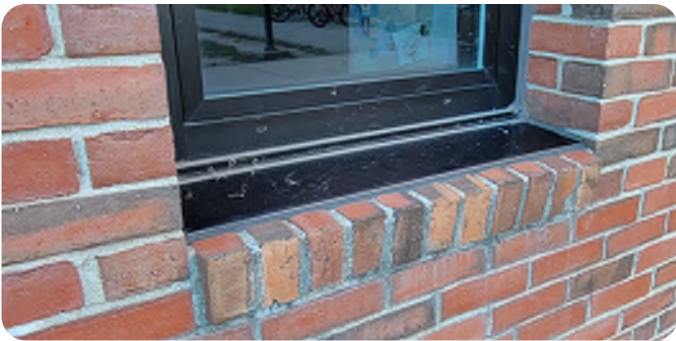
Replacement window with sill extension
