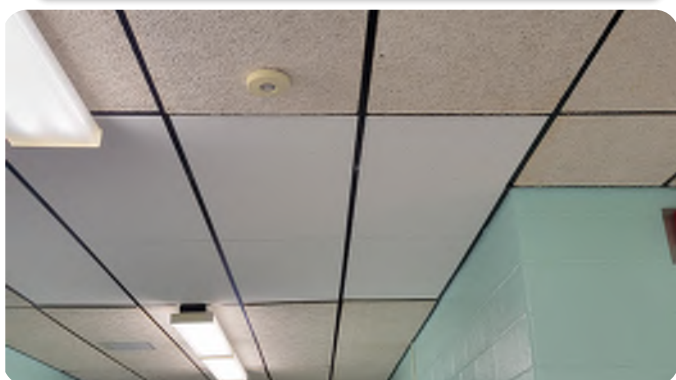
Mix of ACT and “Tectum” ceiling tiles in corridor
