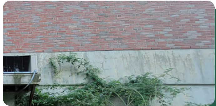
Concrete foundation wall
