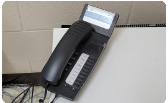
Typical telephone unit in classroom
