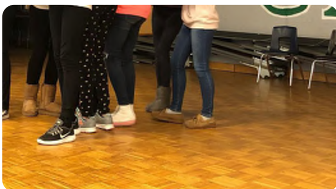
Original parquet stage floor in cafeteria
