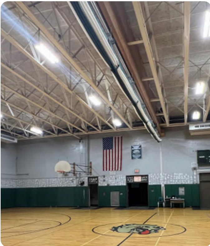
Typical gymnasium roof framing
