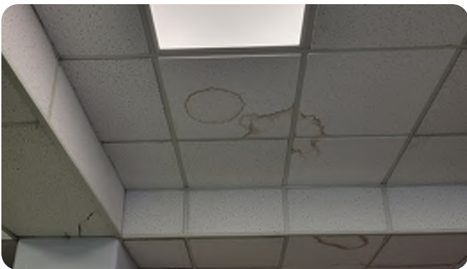
Ceiling in Library
