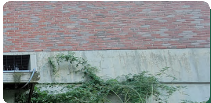
Concrete foundation wall
