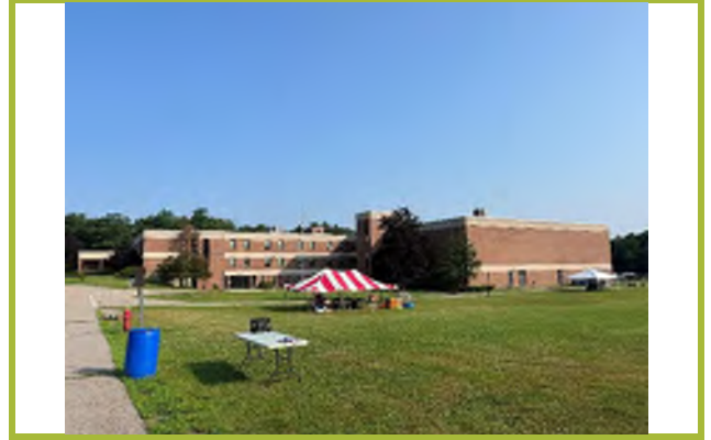
Photograph #2: Southwestern exterior.
