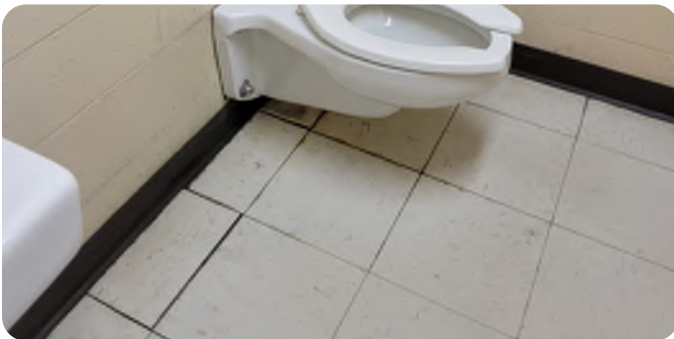
Lifting VAT in toilet room
