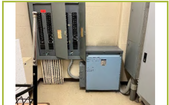
Photograph #22: Elevator machine room.
