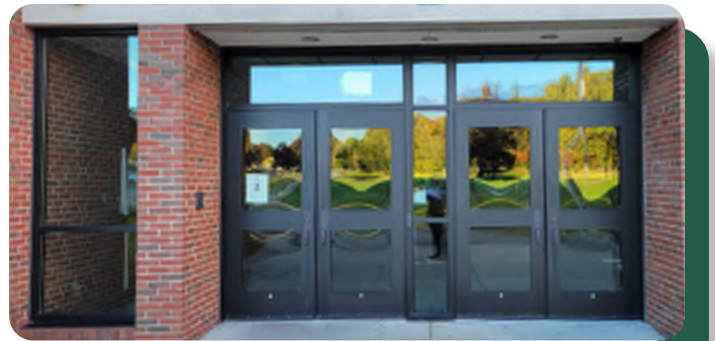
Replacement window and doors at main entrance
