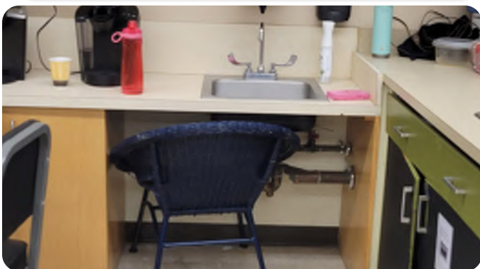
Exposed piping under sink in Life Skills classroom
