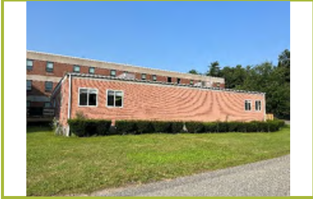
Photograph #7: Daycare to the adjacent northeast of the subject property building.
