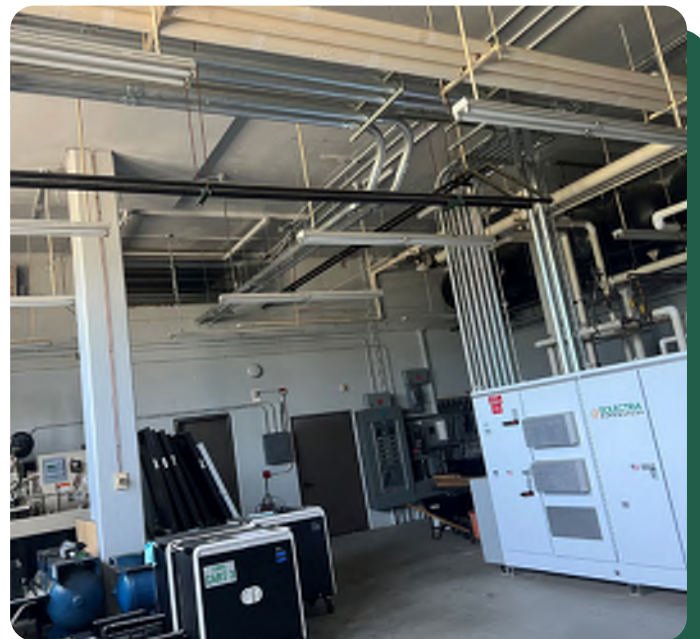
Typical floor slab viewed from Mechanical room
