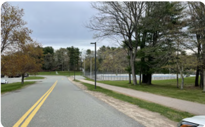
Existing site entrance drive with no curbing
