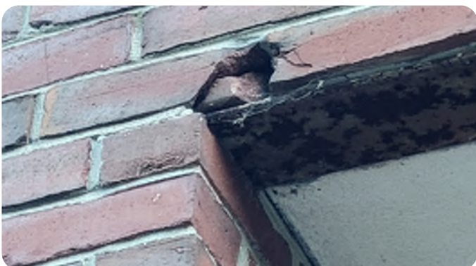
Damaged brick
