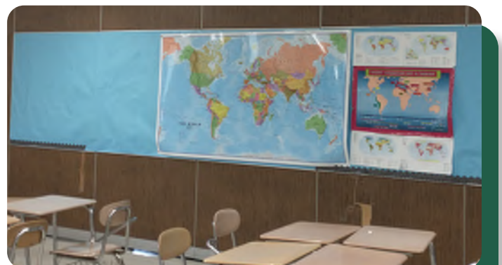
Operable classroom divider with surface damage
