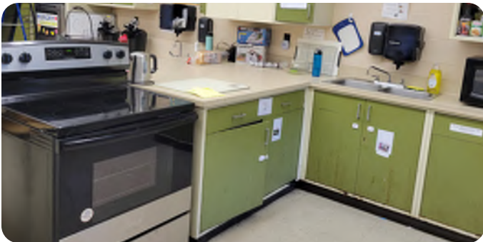
Range controls in Life Skills classroom
