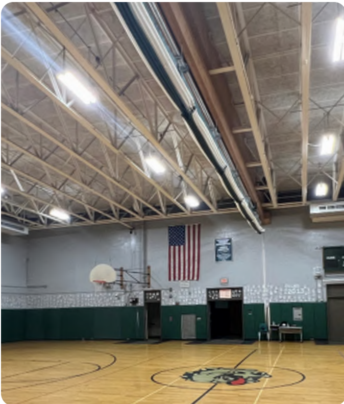
Typical gymnasium roof framing
