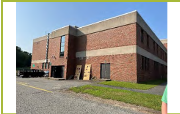
Photograph #3: Northeastern exterior.
