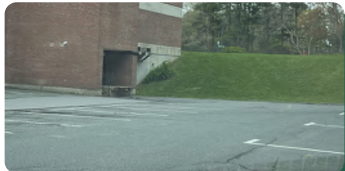
Existing loading area
