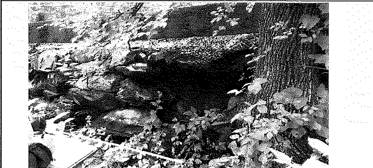
Photo taken July 19, 2021 showing downstream wall west of culvert, missing stones and tree in wall
