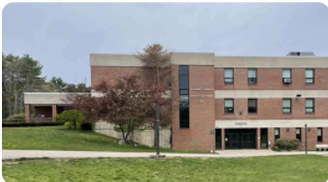
Slope and cross slope at exterior approach to main entrance
