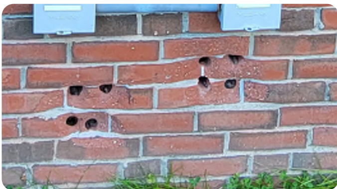
Damaged bricks
