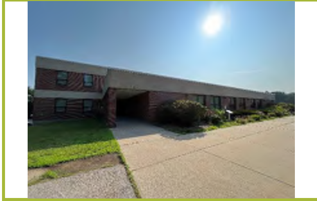
Photograph #1: Southeastern exterior.
