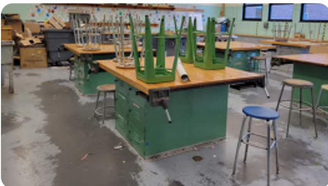
Painted concrete floor in Tech Ed. classroom
