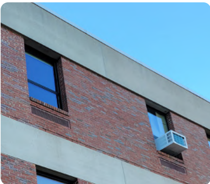
Classroom with unit air conditioner
