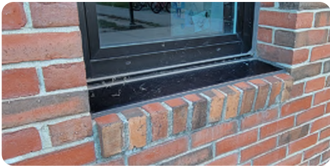
Replacement window with sill extension
