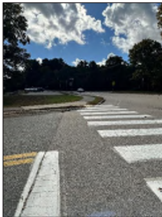
Photo 1. Sight distance looking east (left) from the southern driveway
