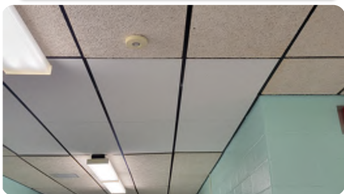
Mix of ACT and "Tectum" ceiling tiles in corridor
