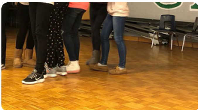
Original parquet stage floor in cafeteria
