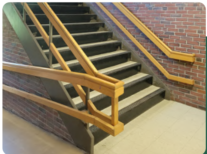
Existing stair railings
